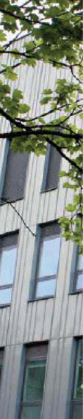
lokfold is a high-quality, fully supported, metal roofing and cladding system available in a variety of quality metal finishes including pre-painted and mill finish aluminium, zinc, copper and micro zinc.
