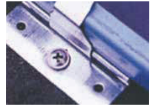
expansion and contraction gap
